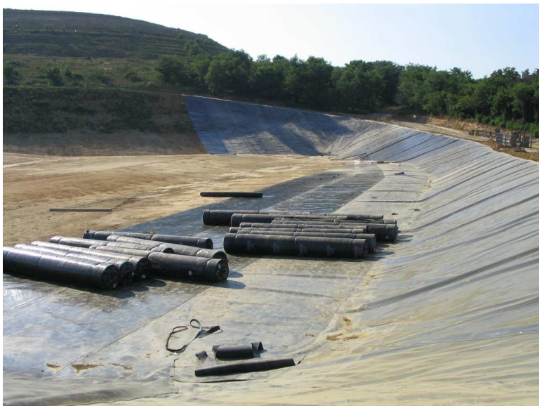
The membrane at the bottom of the new unit.
