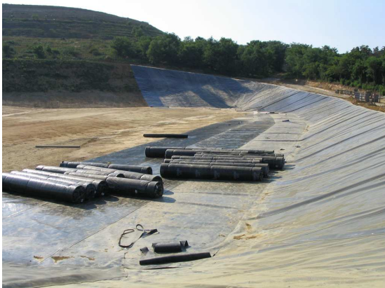
The bottom layer at the new part of the Nagykanizsa landfill and at the background – the old landfill.
