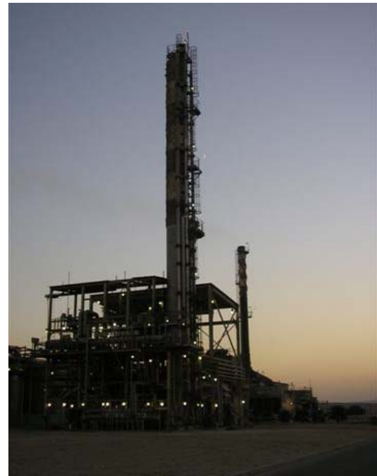
Picture of the N3 plant at Mishor Rotem
