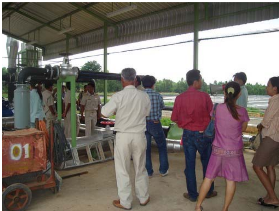
Figure 5: Visitors inspecting the biogas plant
