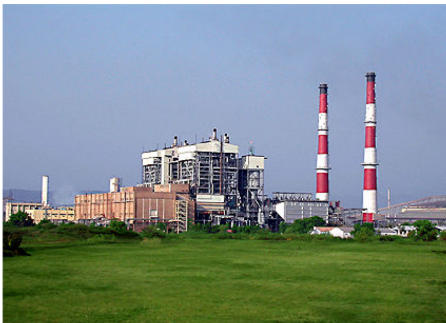
Figure1: JTPCL Site Overview
